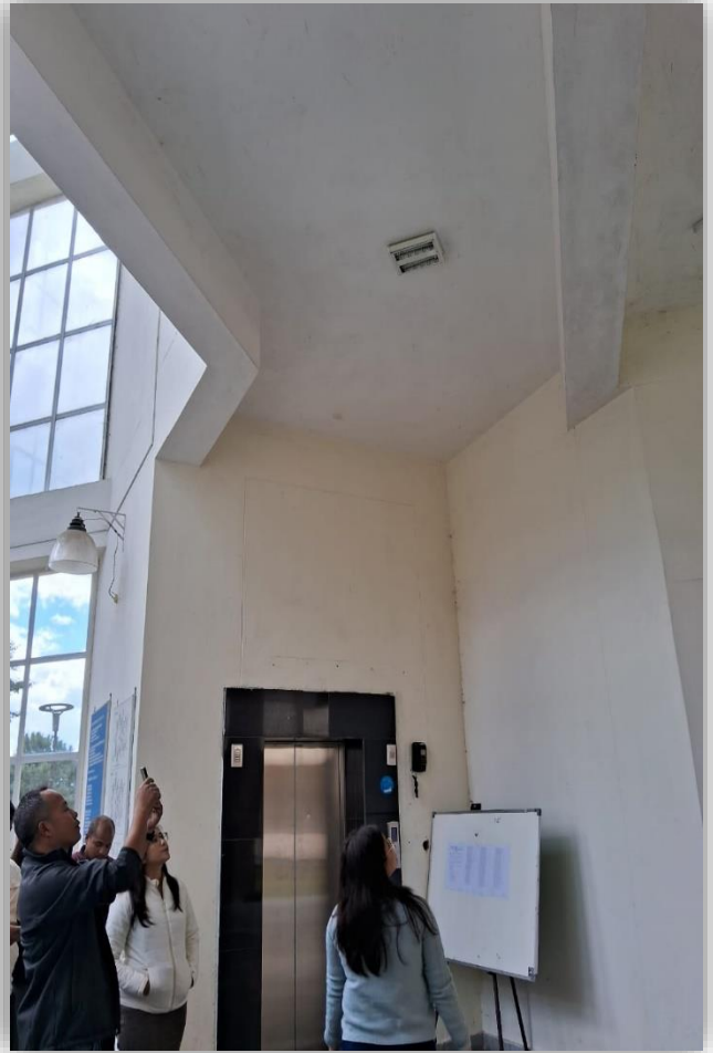
Irregular Joints (should be perpendicular) and Column Joints are not at same angle.
