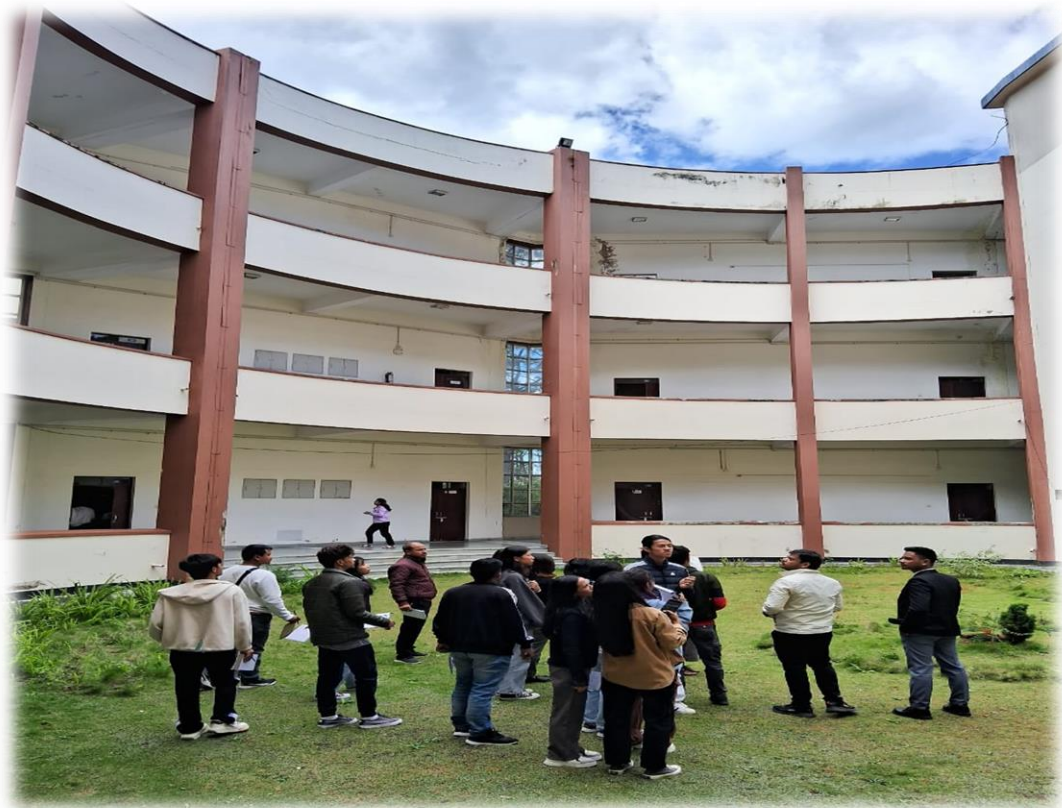
Not Enough Space in the center of the building.
