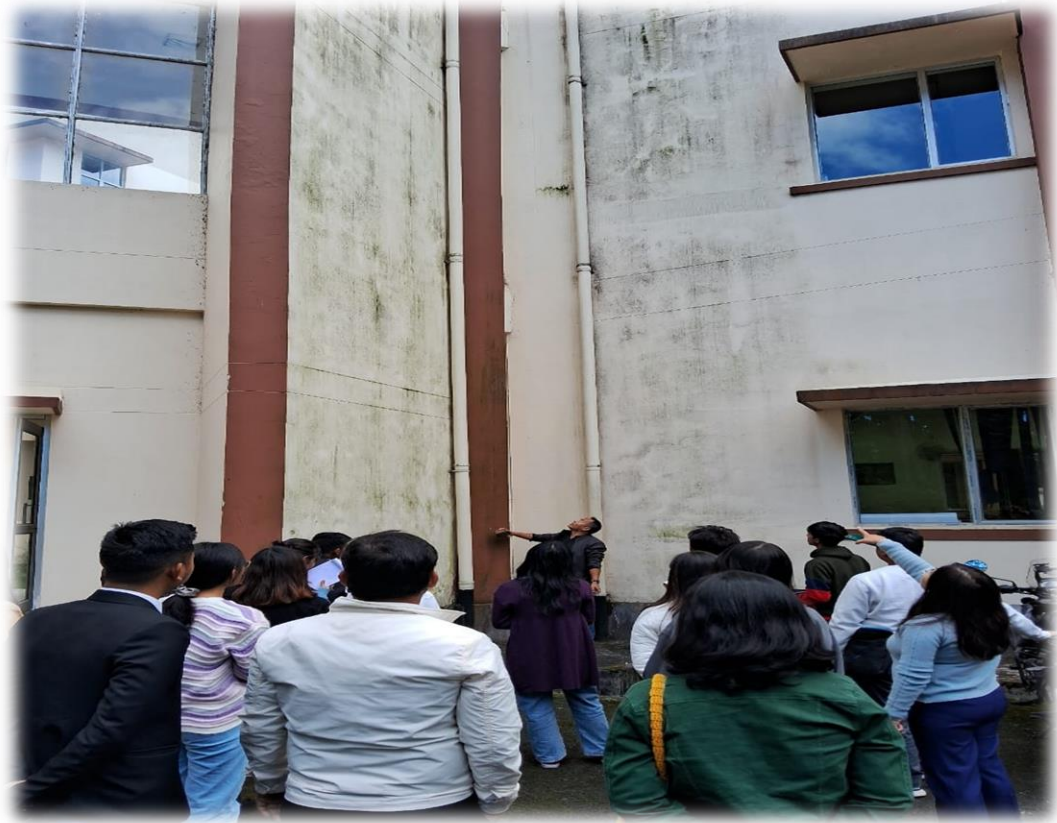
The quality of the concrete is poor.
