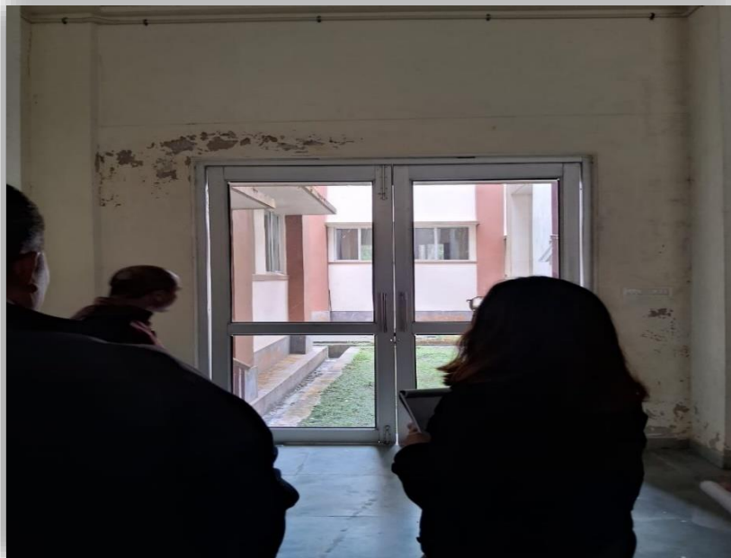
Emergency exits are in the wrong place.
