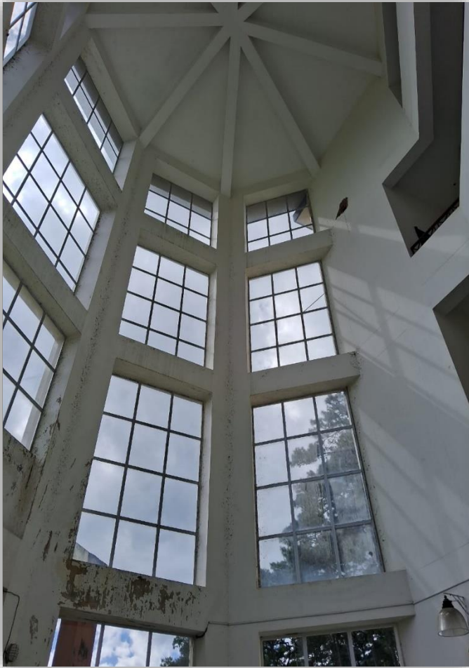
Irregular Joints (should be perpendicular) and Column Joints are not at same angle.
