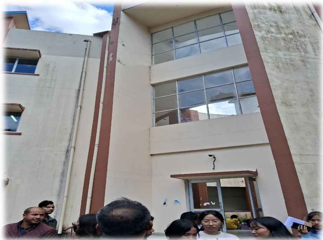
Windowpanes without iron bars.
